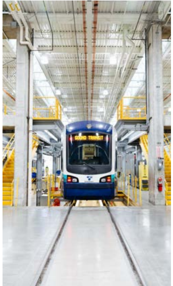
Link light rail trains are parked on maintenance platforms in the Link Maintenance Building.
